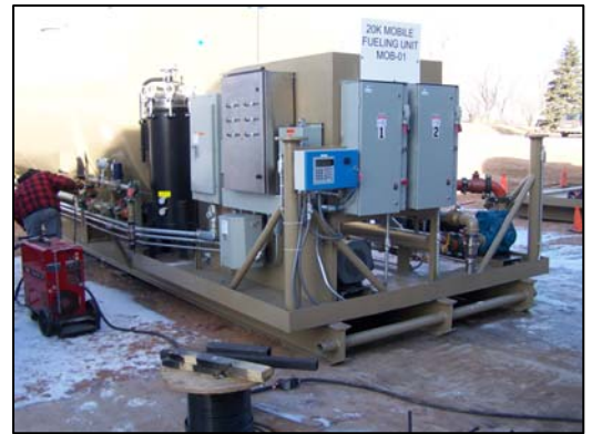
Remove tank from shop and finalize construction of Mobile Fueling Depot
