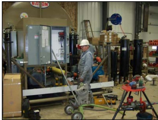
Wire in motors, electric valves, etc.
