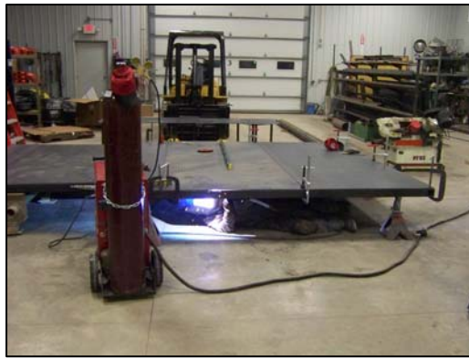
Construct fuel platform for front and back of tank
