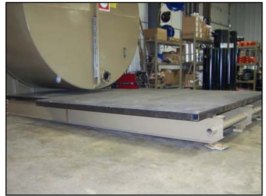
Weld platforms to tank skid
