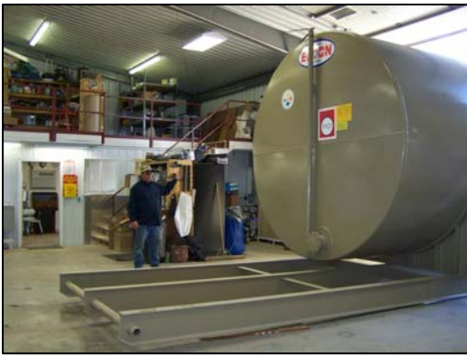
Move tank in to shop
